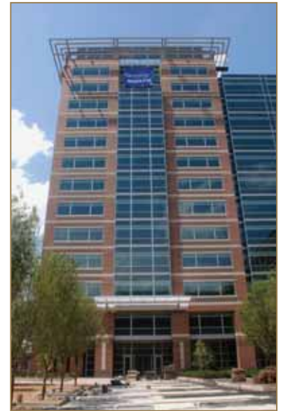
Located in Technology Square, the Centergy Building houses the DSP and telecommunications groups.
