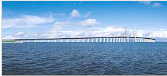
The recently completed Oresund Link Bridge, which crosses the main channel of a 10-mile span of water and small islands between Denmark and Sweden, was designed with the assistance of GT STRUDL. It is the world's longest cable-stayed bridge that carries both rail and vehicle traffic. (300-dpi JPEG version - 663k)
